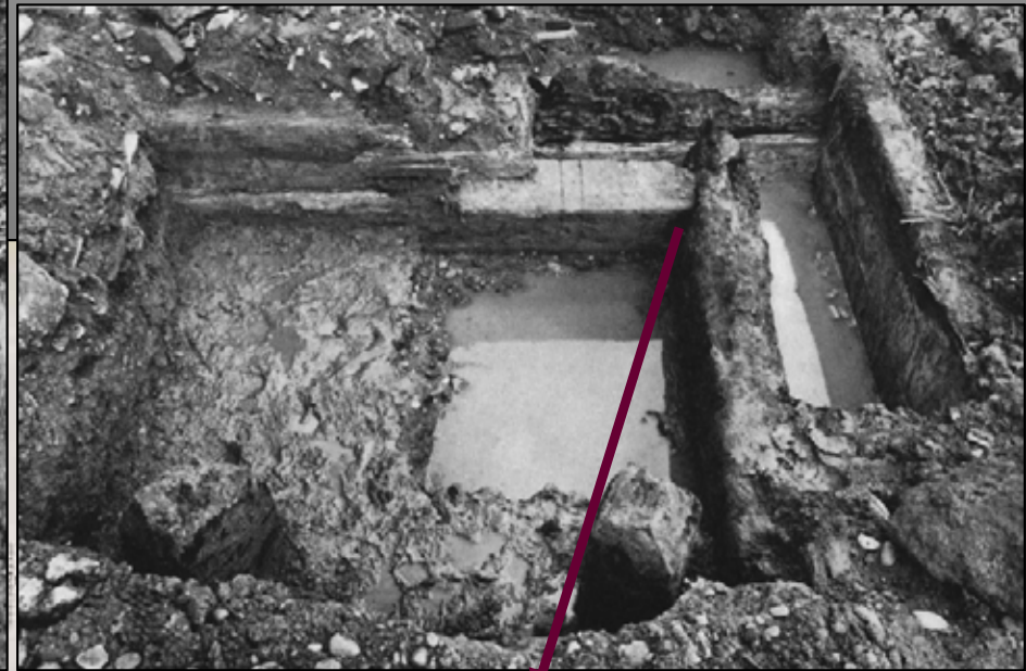
Spundwand an Pfeiler 7
